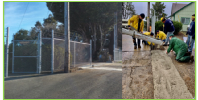
Assisting with Entrance Gate
