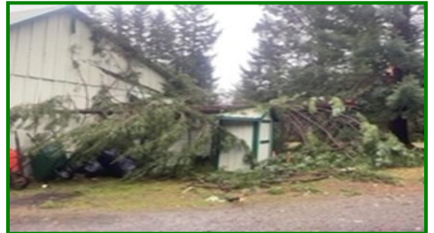
Fourmile Pump House
