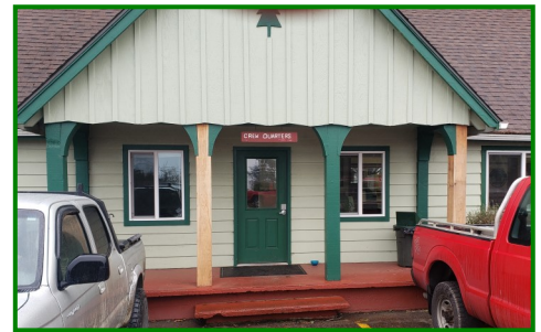
Support Beams on Coos Bay Crewhouse & Warehouse
