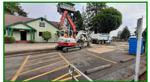
Sewer Line Replacement
